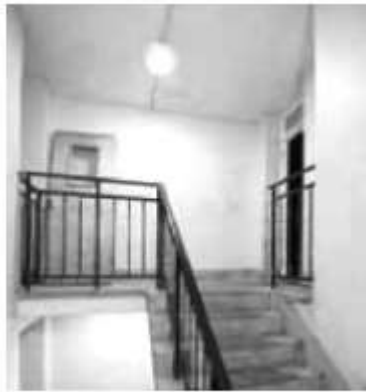
photo of stairwell with LED fitting
