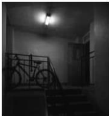
photo of stairwell with fluorescent fitting
